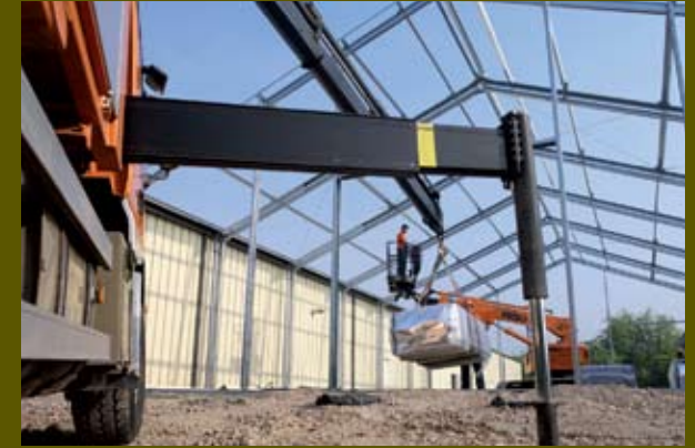
Light but solid. Every part can be manipulated by 2 people. All parts fit together like a giant building kit.
